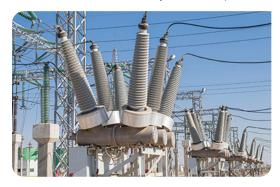
to homes and businesses world-wide. The rapid interruption of electrical power circuits is an essential function, especially in cases of overloads or short circuits when immediate current flow interruption becomes necessary. Circuit breakers perform this function repeatedly, reliably, and quickly.
